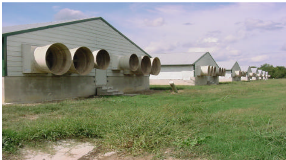
Figure 7.5 CAFO Houses – Rear View
